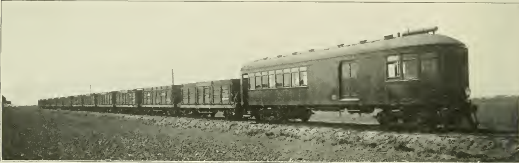
Hall-Scott Gasolene Motor Car Hauling Twelve 20-Ton Beet Cars.
